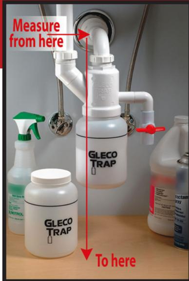
To determine the appropriate size for The Gleco Trap and replacement bottles, measure from the vertical center of the waste line to the floor.
