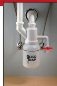
Place extra bottle (or container) that can hold at least 30 ounce of water underneath the arm on the right. Open valve to drain water at the top of The Gleco Trap. **DON'T FORGET** to turn valve into off position again. Unscrew the used bottle and replace it with another bottle or even the reuse the same bottle after disposing of the contents properly.
